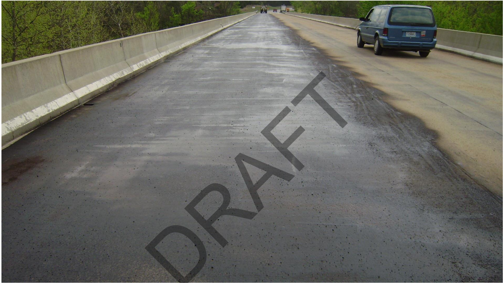
Typical bridge deck seal
