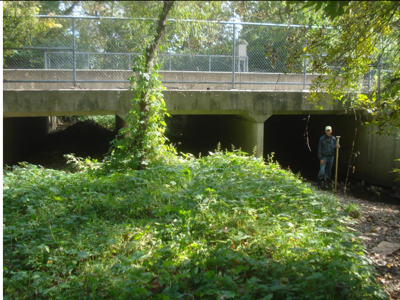
Two of the three box culverts beneath Kingsland Ave. on Engelholm Creek are severely clogged by a sand bar and overlying vegetation. Note USGS gauging station 07010035 near the bridge deck in the upper right center of the photo. Photo date Oct 20, 2019.
