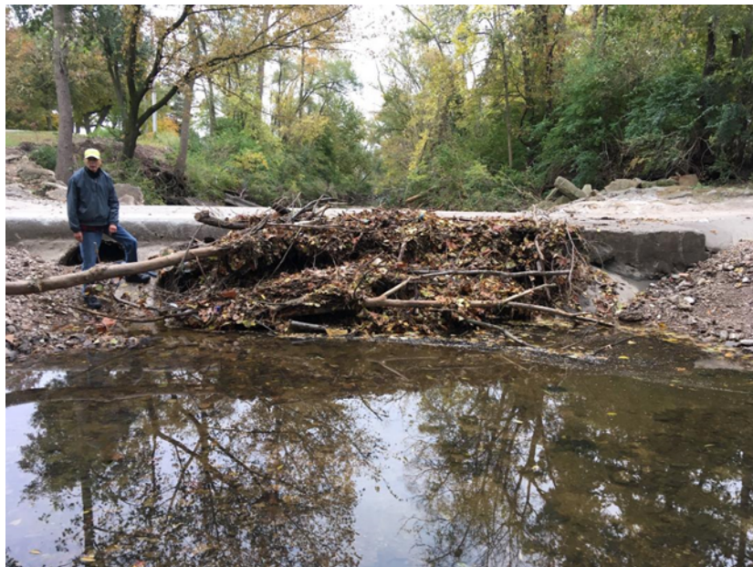
Low water crossing as in photo 5, taken three days later showing blocked culverts after elevated streamflow on October 26. Photo date October 28, 2019.
