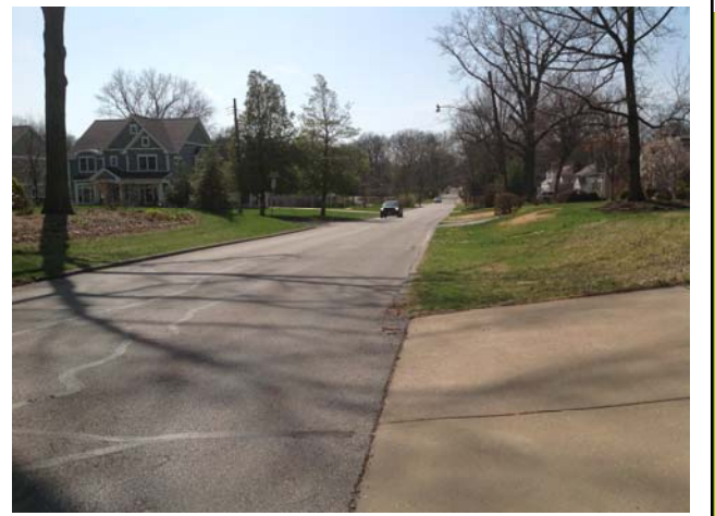
Photo - #4 No sidewalk, rutting in wheel path
