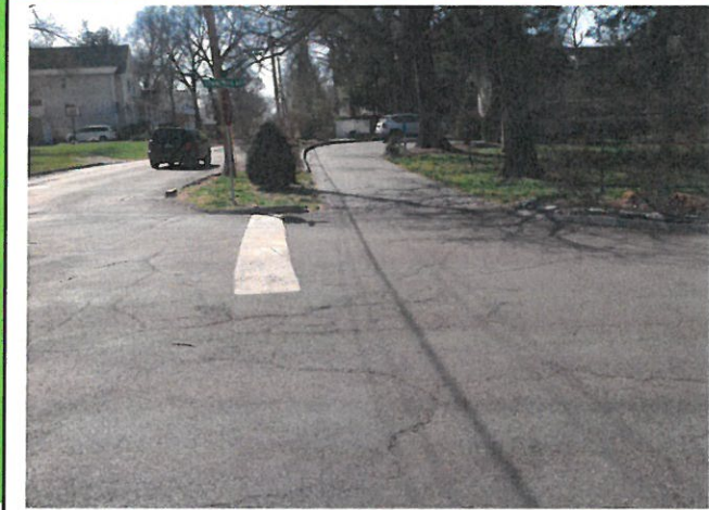
Moderate cracking.
