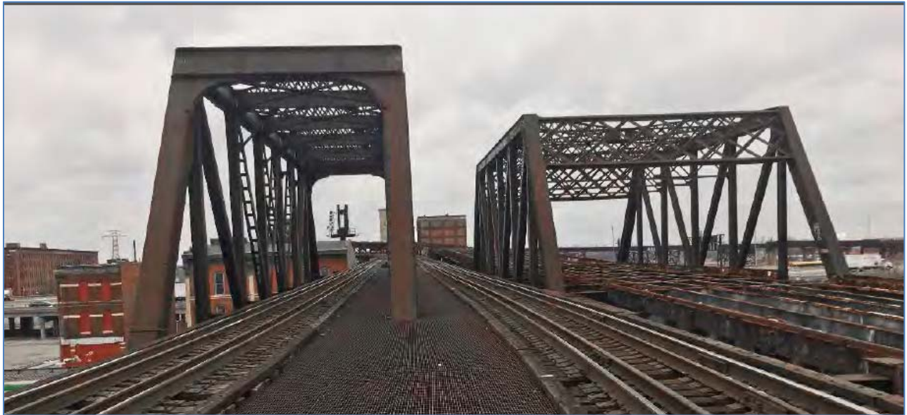
Figure 2 -- Replacement of Existing Trusses
