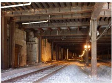
**Union Station Tunnel Rehabilitation.** *St. Louis, MO* | MM is providing Phase I, II, and III engineering services to reconstruct the steel portion of the tunnel. MM is collaborating with the Owner and Contractor to deliver the project using the CM/GC project delivery method and working to find ways to reduce cost. MM is providing engineering services for temporary construction access and temporary works as required, as well as answering RFI's, and reviewing shop drawings.
