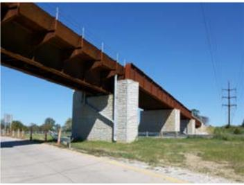
**Columbia Terminal Railroad US Highway 63 Overpass. *Columbia, MO*** | MM designed the overpass structure, a six-span steel girder bridge with four deck girder approach spans and two 85-foot through plate girder main spans. Design was originally planned to take sixteen months, however, due to the unexpected availability of Federal funding, the design phase was expedited and **compressed by six months**.
