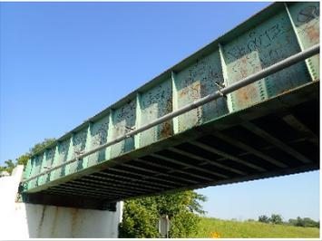
**CSX Railroad Over Scott Troy Road Emergency Inspection.** *O'Fallon, IL* MM performed a structural inspection of the entire bridge, paying special attention to the impact damage caused by a boom truck striking the north side. The inspection included measuring displacement of the girders due to impact, measuring lengths and magnitudes of cracks and tears throughout the steel members, and performing a visual inspection of the entire structure for deficiencies not related to the impact.
