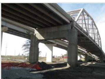
**MLK Bridge Ramp Replacement.** *East St. Louis, IL* | Phase I, II and III engineering services are being provided for the replacement of the original approach ramp structure and miscellaneous repairs to six other structures. Services include overall project management, the preparation of a Bridge Condition Report, Project Report, Type, Size and Location plans, Structure Geotechnical Report, Plan Development Outline, final structure plans, and construction services as requested.
