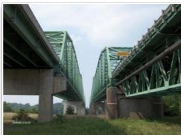
**US 40 Over Missouri River Study.** *St. Charles, MO* | MM assisted with preliminary engineering studies for a new crossing, including locating the preferred alignment for the new crossing, investigating viable structures for both the main river bridge and the approach structures, and providing tie-ins to the existing highway network. Adequate clearance for construction, inspection and maintenance, progressive collapse, and site restrictions were also investigated.
