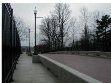
**Mississippi Avenue Bridge Replacement.** *Crystal City, MO* | MM designed this replacement structure while accommodating the increased vertical clearance requirements of BNSF. In order to achieve the required clearance while minimizing the effect on the approach roadway, MM designed the structure with a two-foot superstructure depth. Aesthetic features were also included in the design to compliment the downtown business district.
