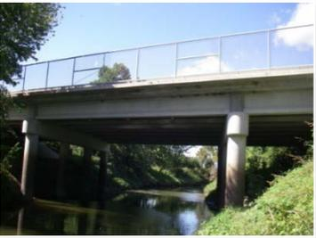
**Creve Coeur Mill Road Bridge No. 232 over Fee Fee Creek.** *Maryland Heights, MO* | Deterioration of the end diaphragms and adjacent girder ends developed in this bridge. MM provided an in-depth inspection and structural investigation and found various structural constraints were inducing tensile stresses into the girder ends / integral end bents causing cracking. A rehabilitation strategy was proposed to eliminate these constraints and final plans and specifications were provided.
