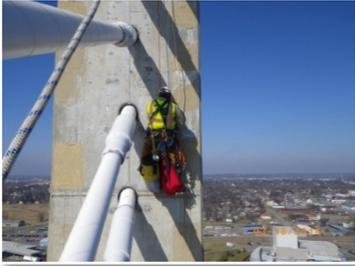
**Bill Emerson Memorial Bridge Inspection.** *Cape Girardeau, MO* | MM was selected by MoDOT to perform the 2014 NBIS and FCM inspections of the bridge as well as the first in-depth inspection of the structure's complex features. MM provided a complete "hands-on" visual and tactile inspection of each cable, including anchorages, utilizing technical access inspection methods. Vibration testing of the cables and ultrasonic testing of the back span hold-down pins were also performed.
