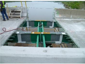
**Interstate 80 Over the Mississippi River Emergency Repairs. *LeClaire, IL*** | IDOT discovered cracks in the top flanges of various cantilevered floorbeams during a routine inspection. Rehabilitation details were developed to correct the fatigue prone details and prevent future cracking. MM worked under an extremely **compressed design schedule of four months** to allow construction to begin as soon as possible to restore full traffic to this structure.
