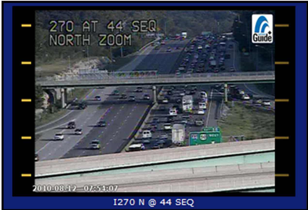
Figure 4: Northbound I-270 Congestion to I-44 (Morning)
