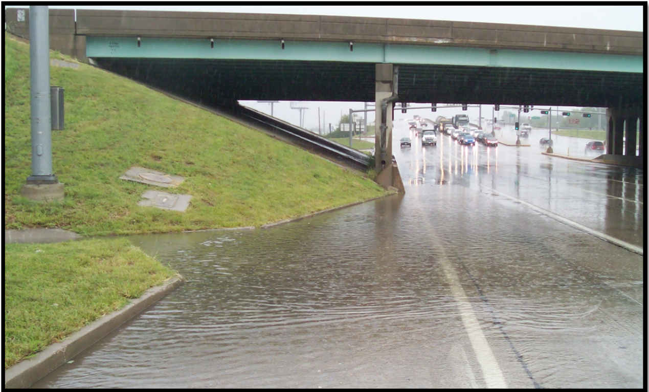
Figure 18: Local Flooding Event at I-44 / Route 141 Interchange (Looking North, 2010)
