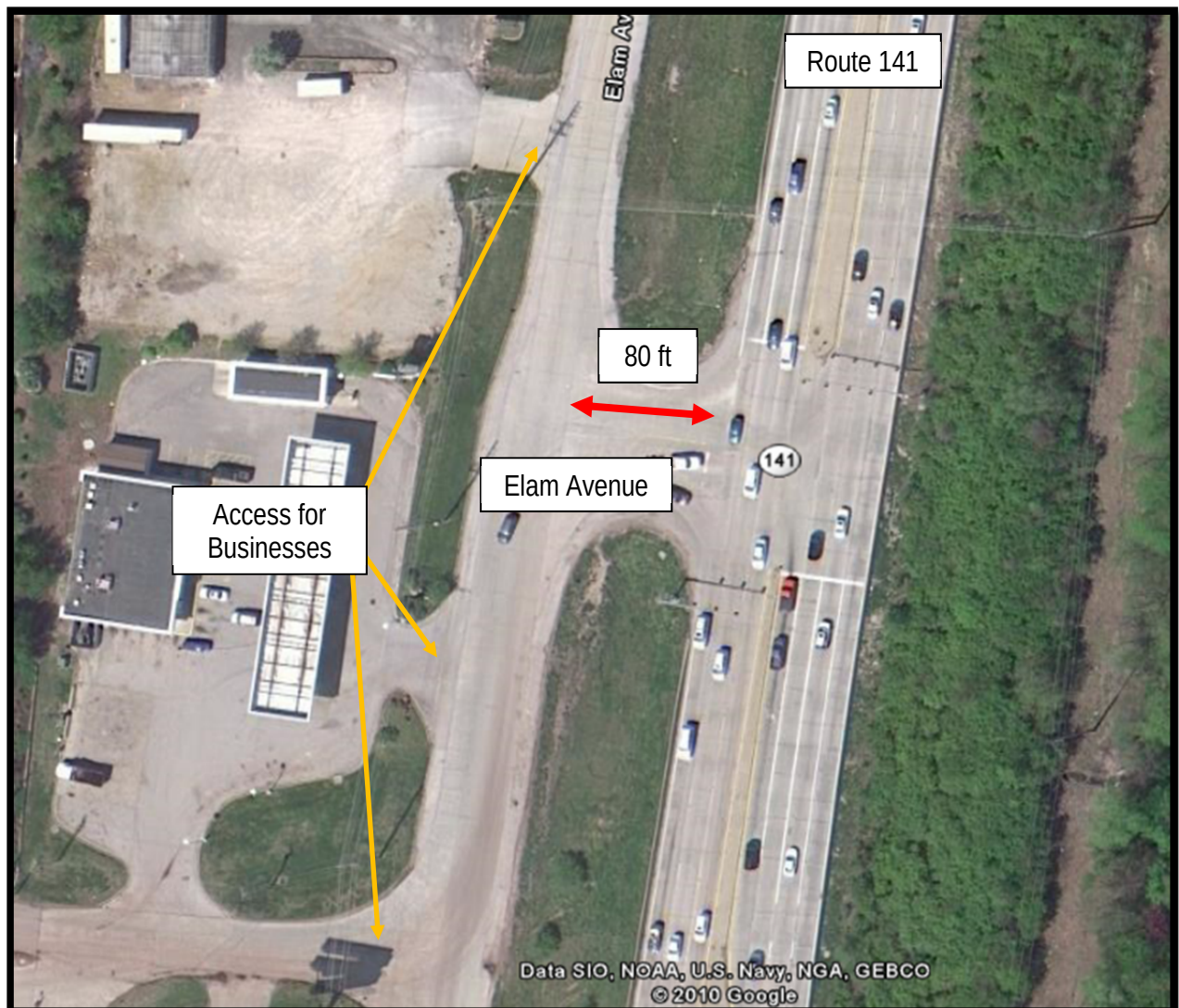
Figure 10: Route 141 at Elam Avenue
