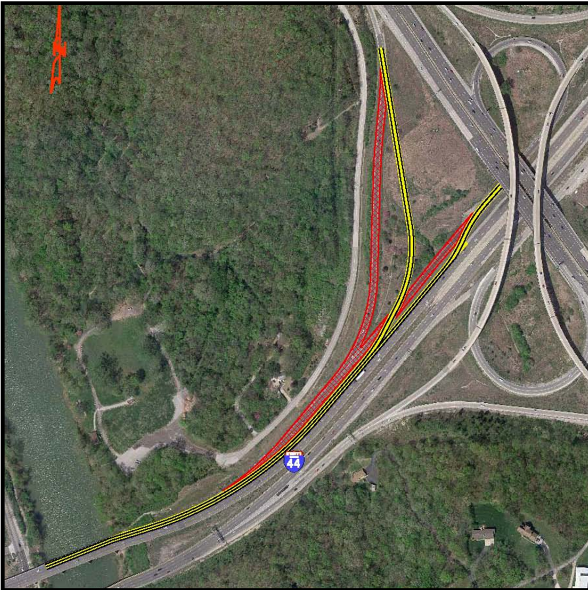
Figure 42: Relocated Southbound I-270 to Westbound I-44 Ramp
