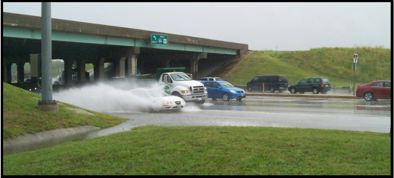
Figure 19: Local Flooding Event at I-44 / Route 141 Interchange (Looking East, 2010)
