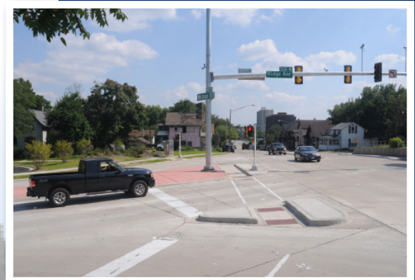
Ridge Avenue/Whitman Street Intersection Improvements Rockford, IL
