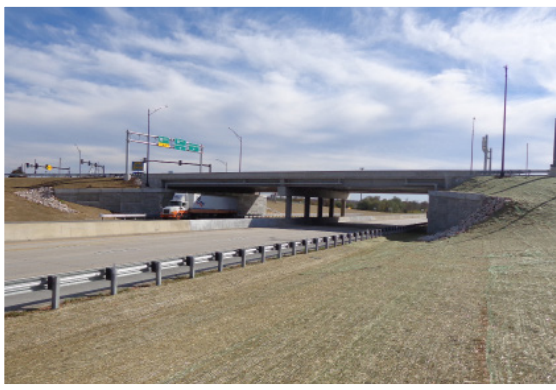
Battlefield Road over Route 65 Interchange Greene County, MO
