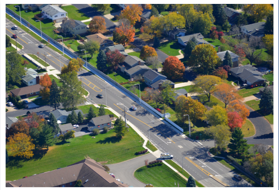
Northmoor Road Improvements Peoria, IL
