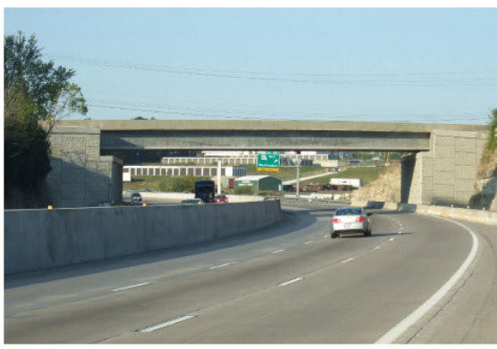
Route 100 over I-44 Franklin County, MO
