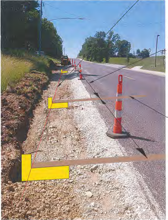
METHOD FOR ESTABLISHING ELEVATION OF CURB NO SCALE
