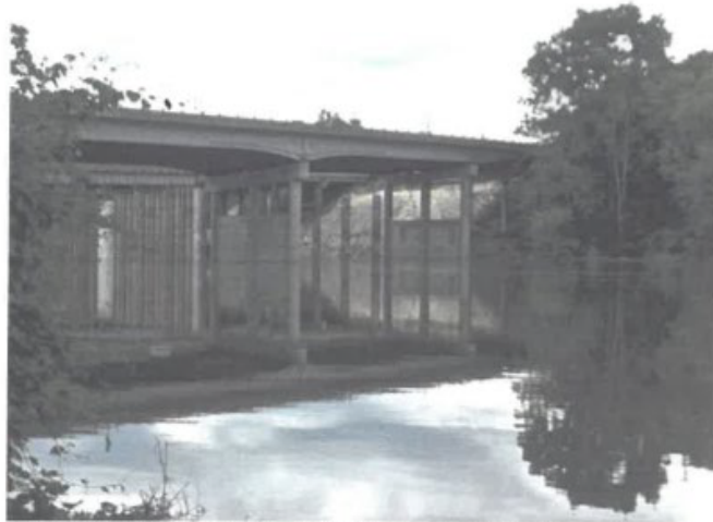
Trail spur/"river overlook" site at 20 ft "moderate" flooding on 5/25/19. The river crested at 44.5 ft in 2015.
