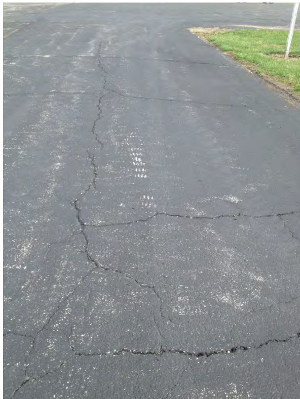
Figures 2 and 3: Block Cracking
