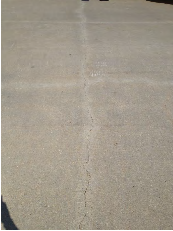
Figures 12 and 13: Linear Cracking
