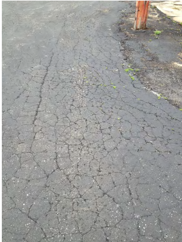
Figures 8 and 9: Fatigue Cracking
