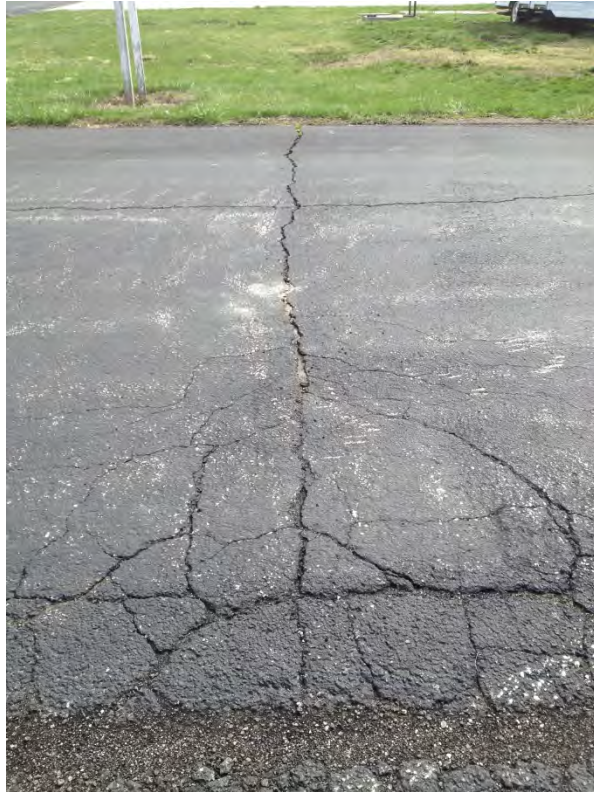
Figures 4 and 5: Transverse Cracking w/ Related Deterioration
