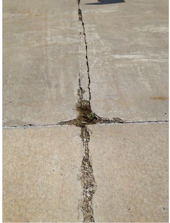
Figures 12 and 13: Linear Cracking
