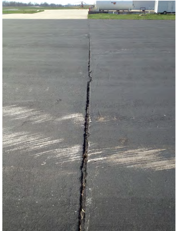
Figures 6 and 7: Longitudinal Cracking
