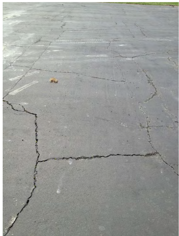
Figures 2 and 3: Block Cracking
