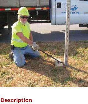
This innovative tool uses a bent piece of round steel rod to level sign bases. It can be operated by hand or foot pressure.
