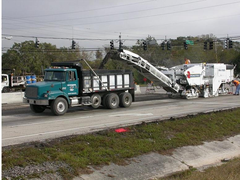
**Figure D-4. Asphalt milling machine and dump trailer**
