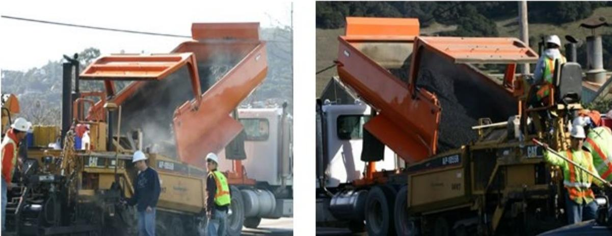
**Figure D-3. (a) HMA placement (b) WMA placement (11)**
