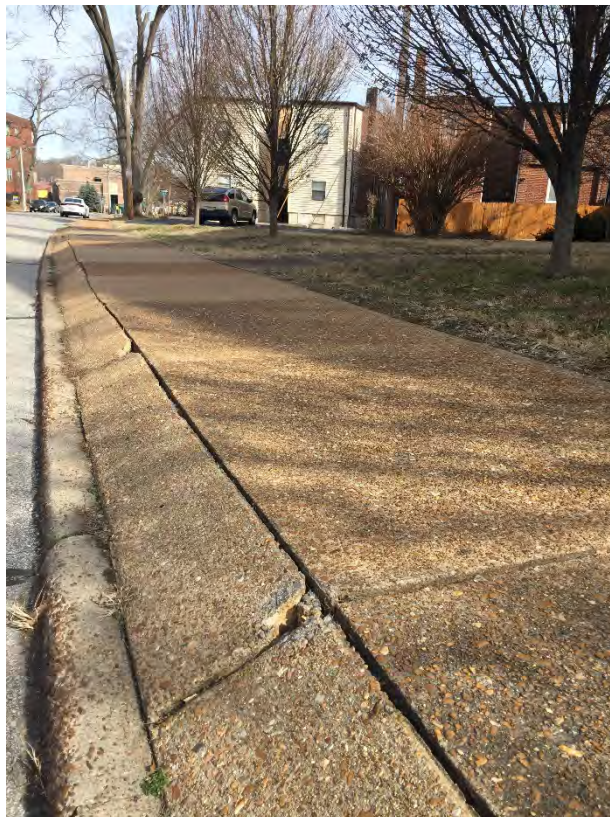
Photo 8: Typical sidewalk section at ground level. Cross slope to steep to be ADA compliant.
