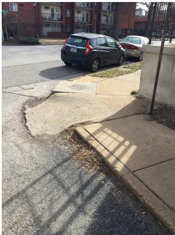
Photo 10: Non ADA compliant curb ramp at Parkview Place Apartments due to proximity to inlet.
