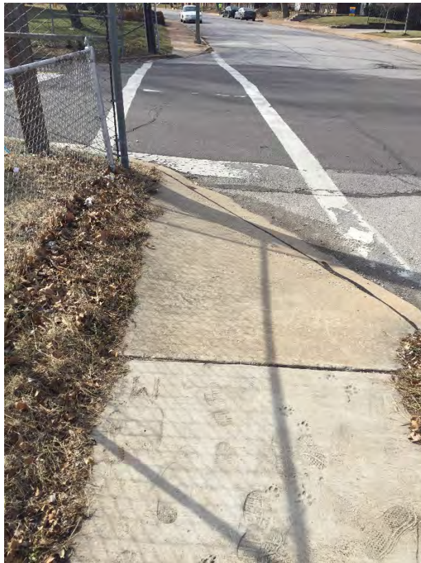
Photo 6: Non ADA compliant curb ramp at Vernon Avenue.
