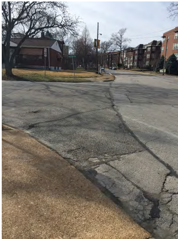
Photo 4: Nonexistent crosswalk pavement markings crossing North Drive.
