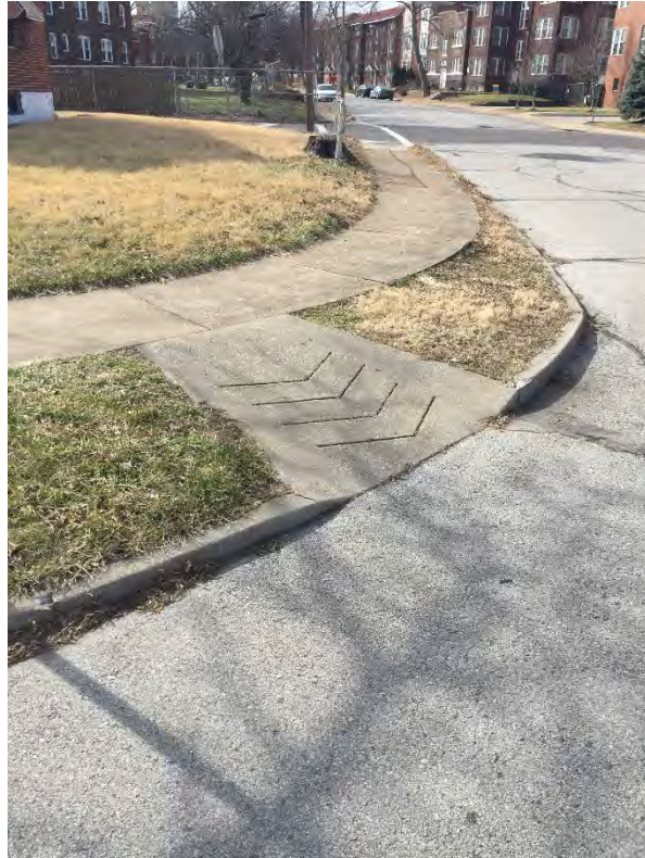
Photo 5: Additional non ADA compliant curb ramp at North Drive.
