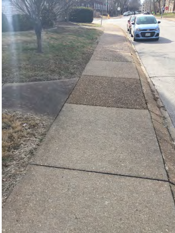
Photo 7: Typical sidewalk section at eye-view. Cross slope to steep to be ADA compliant.
