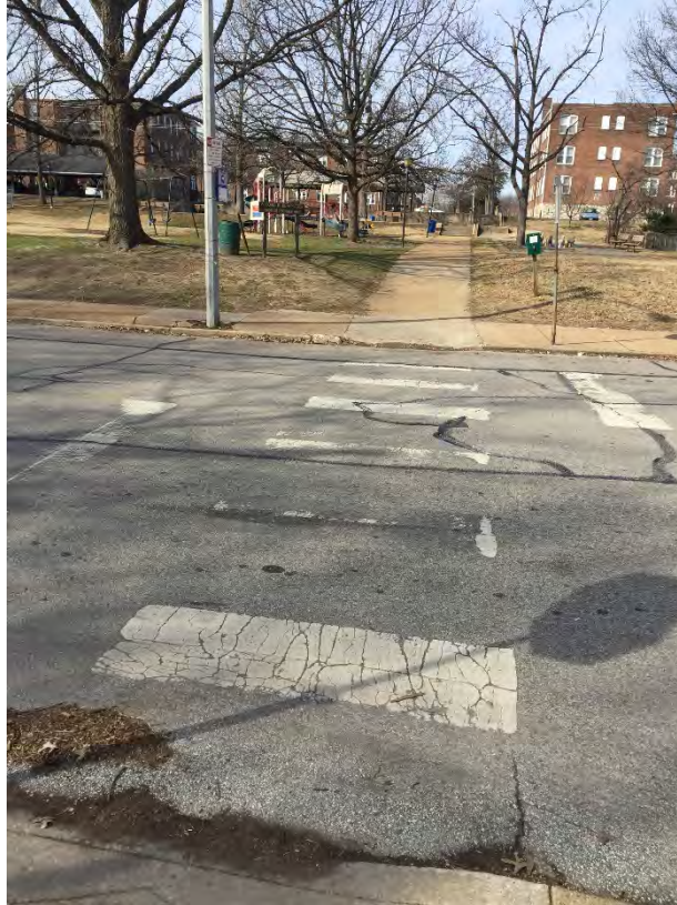
Photo 9: Deteriorated crosswalk and stop bar pavement markings in front of Ackert Park
