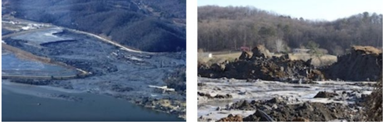
Figure 1.2: A failed impoundment at the Kingston plant in eastern Tennessee [20].
