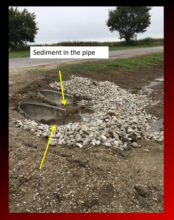
Should consider a BMP between the rock liner and concrete ditch
