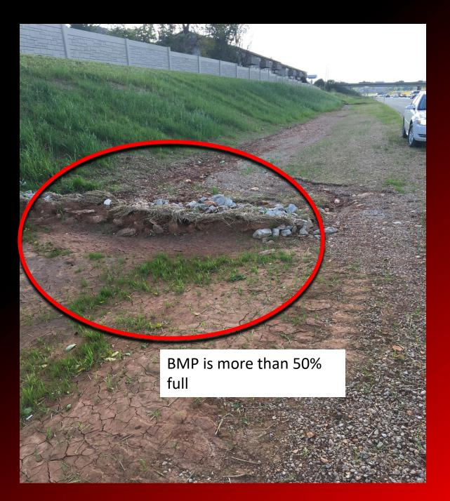
Text book sediment movement in the ditch – cause: insufficient number of BMPs in ditch
