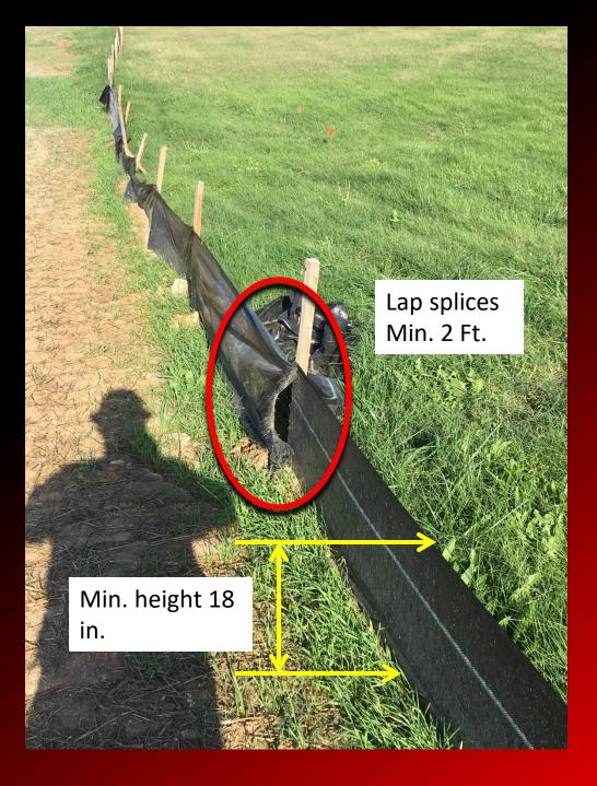
Washout erosion from lack of maintenance to BMP
