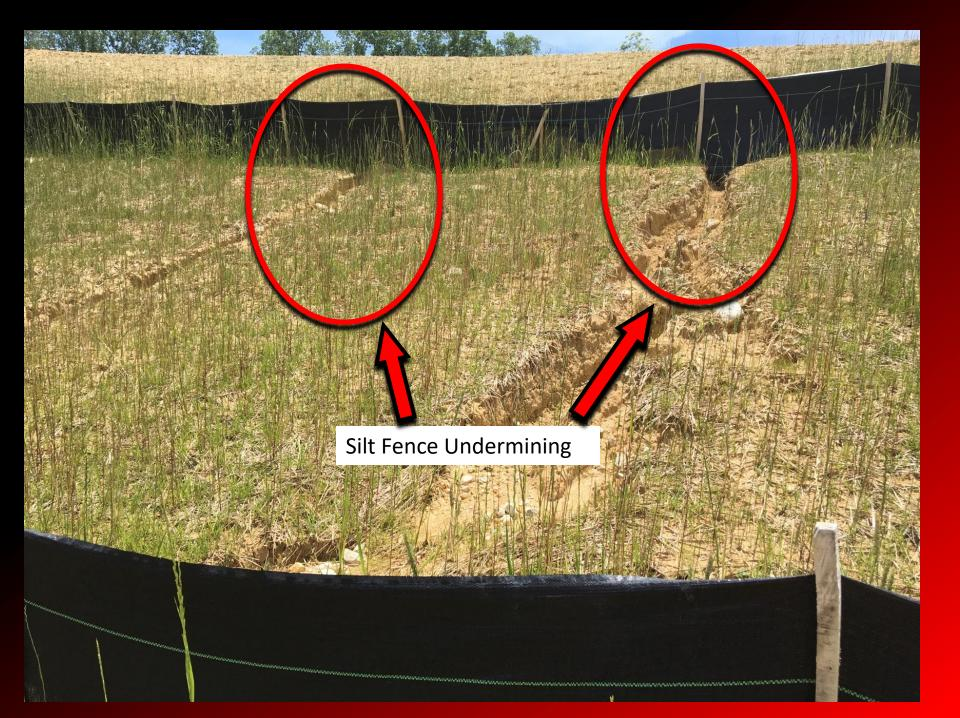
Placing Down stream BMPs only - not sufficient for compliance
