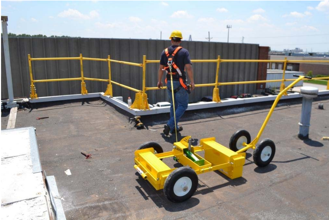
Stinger Cart – 1 person in Fall Arrest, 1 in Restraint
