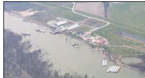
Figure A-9: Pemiscot County Port Authority
