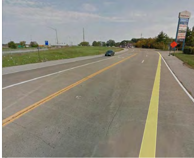
Typical Bus Stop: No shelter, no crosswalk, no sidewalk
