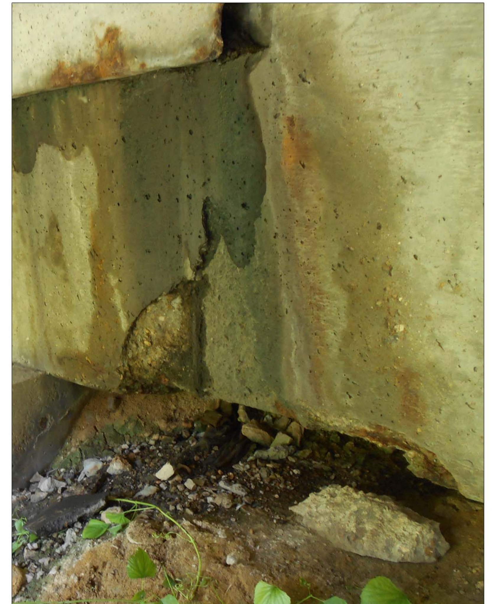
Water seeps through cracks in the roadway above and deteriorates the foundations.
