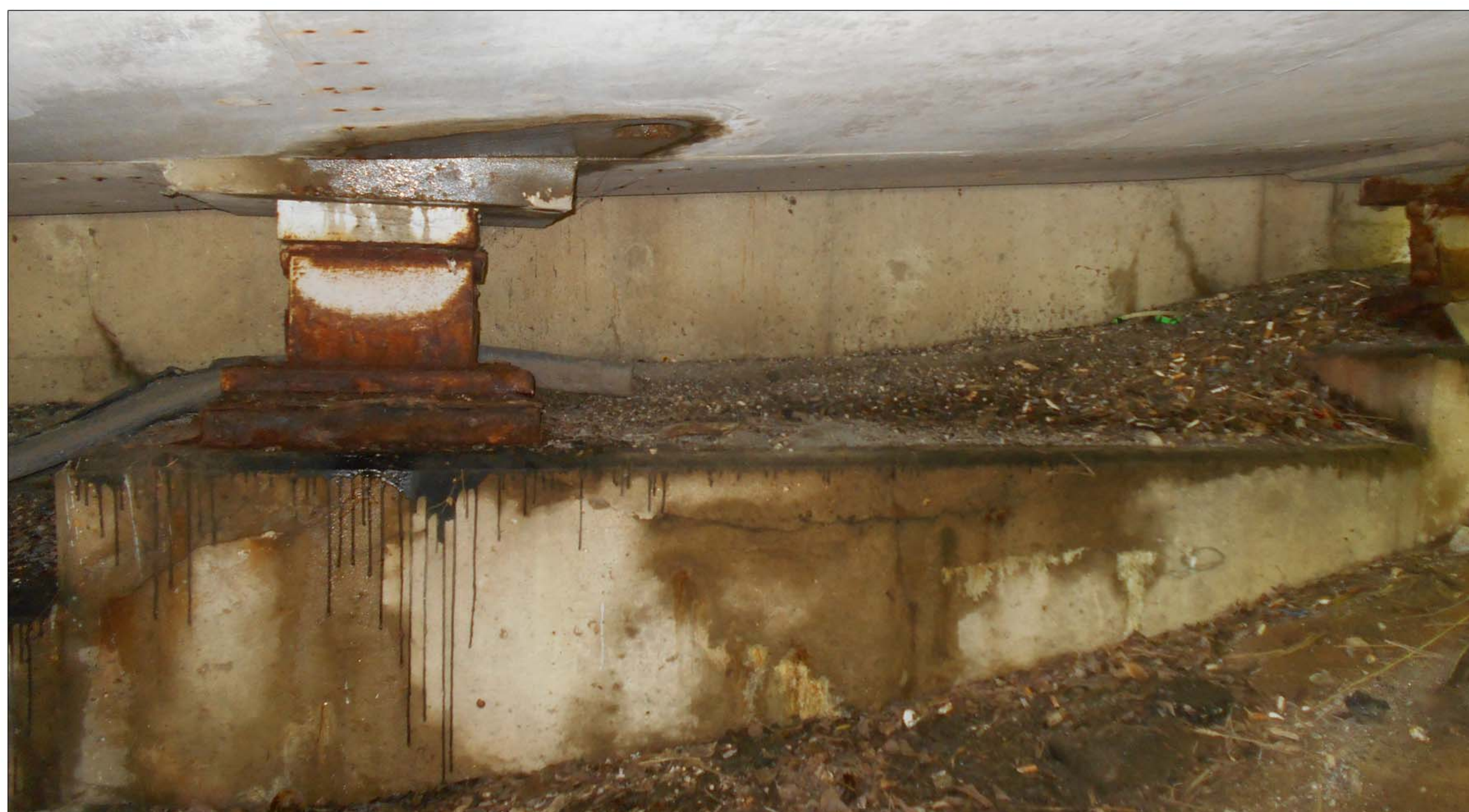
A picture of a rusty bridge support from the side.
