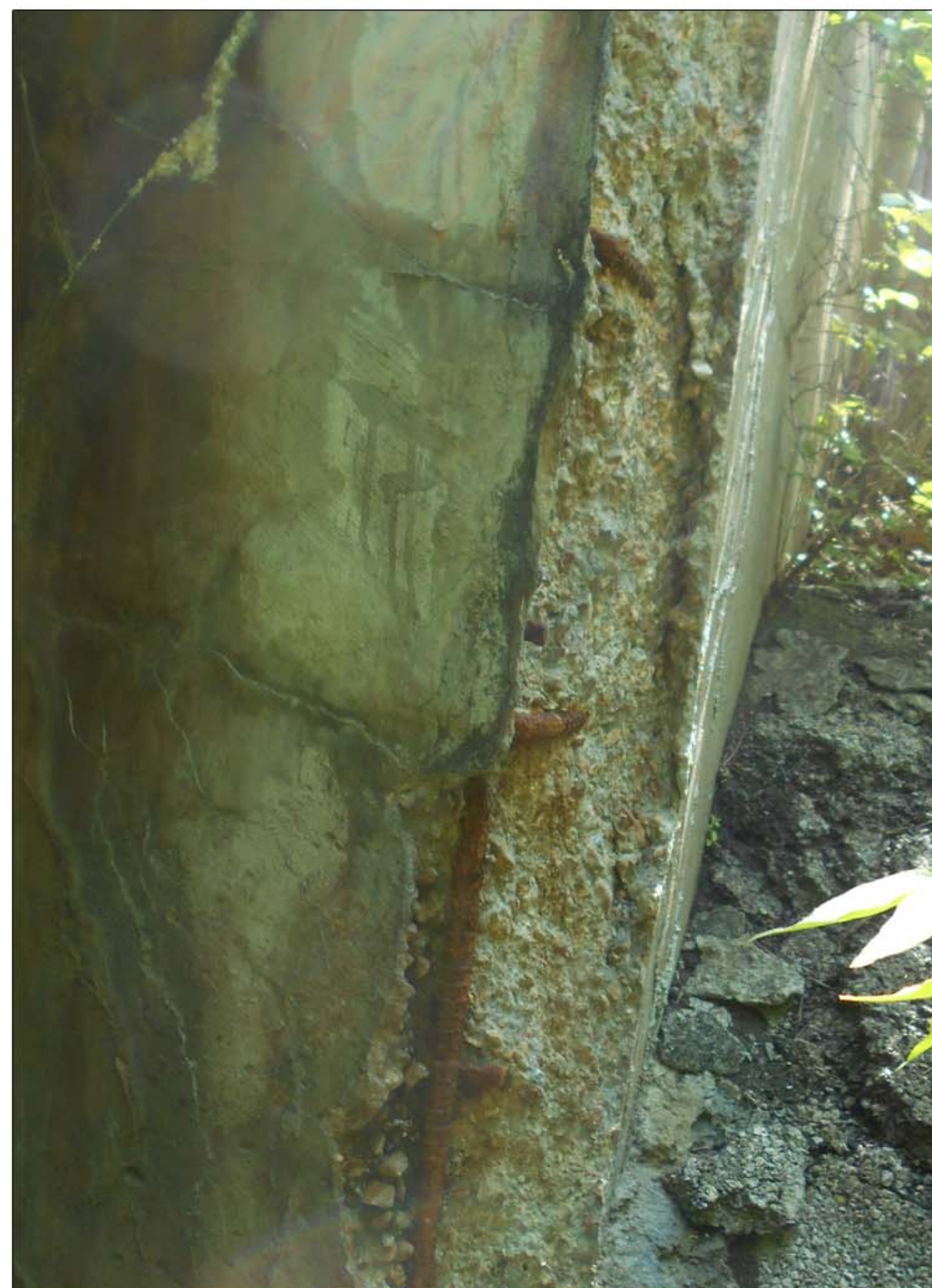
Concrete foundations are cracking and crumbling.
