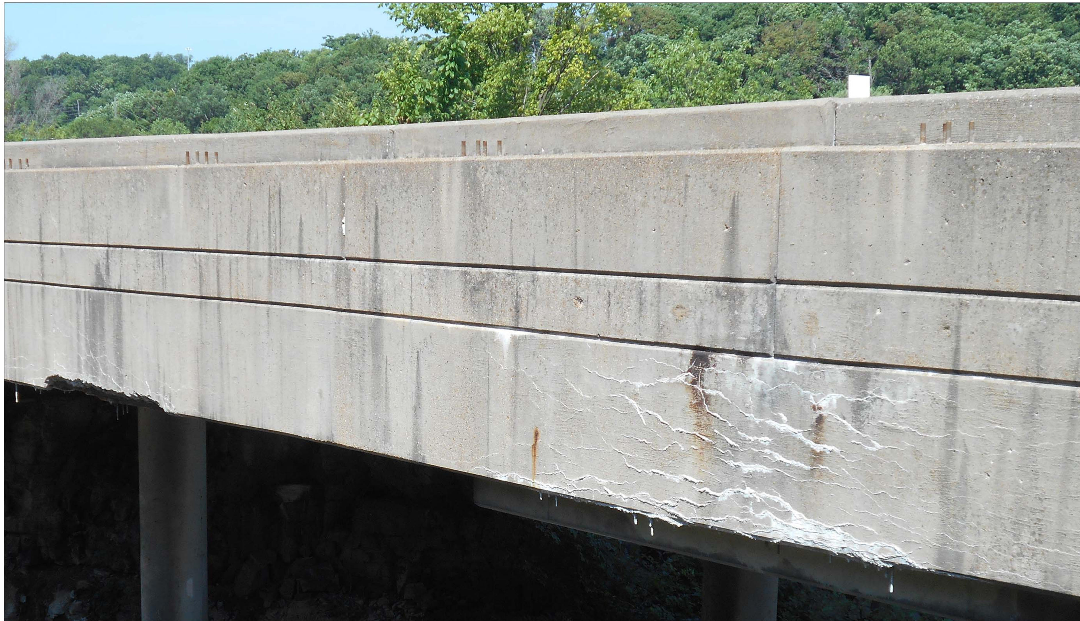
Concrete along the bridges are cracking and crumbling.
