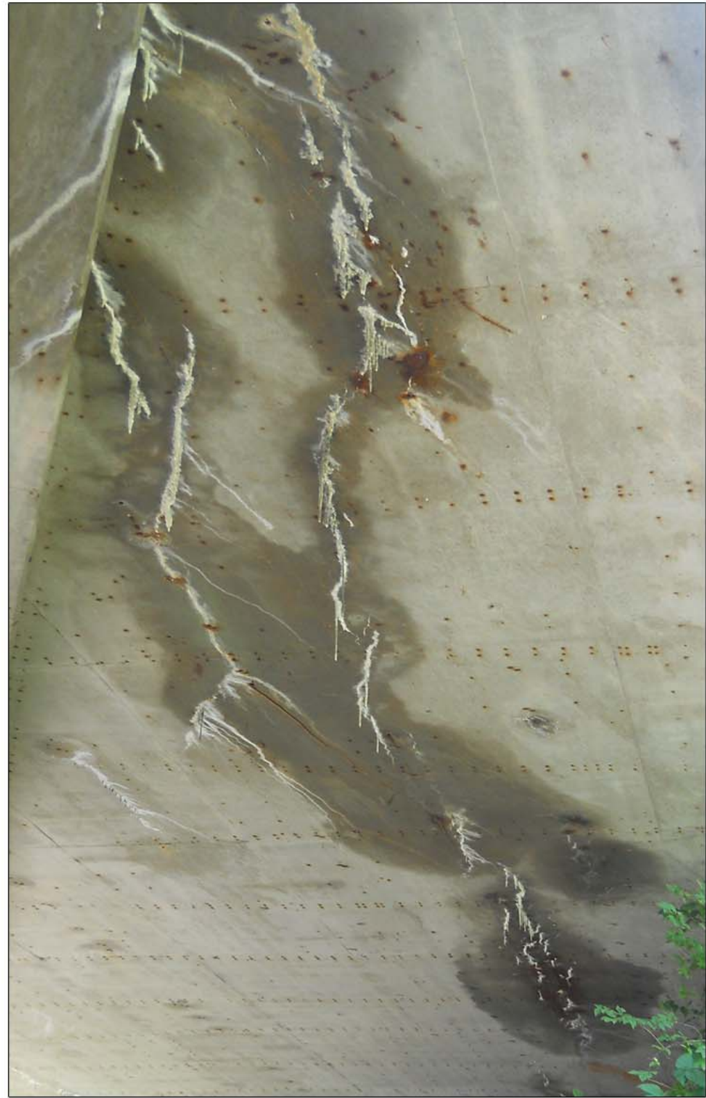
Water seeps through cracks and crevices, breaking down the concrete. In winter, chemicals placed on the road further deteriorates bridges.
