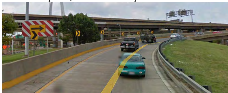
Photo 14: Sharp horizontal curve on Ramp A
