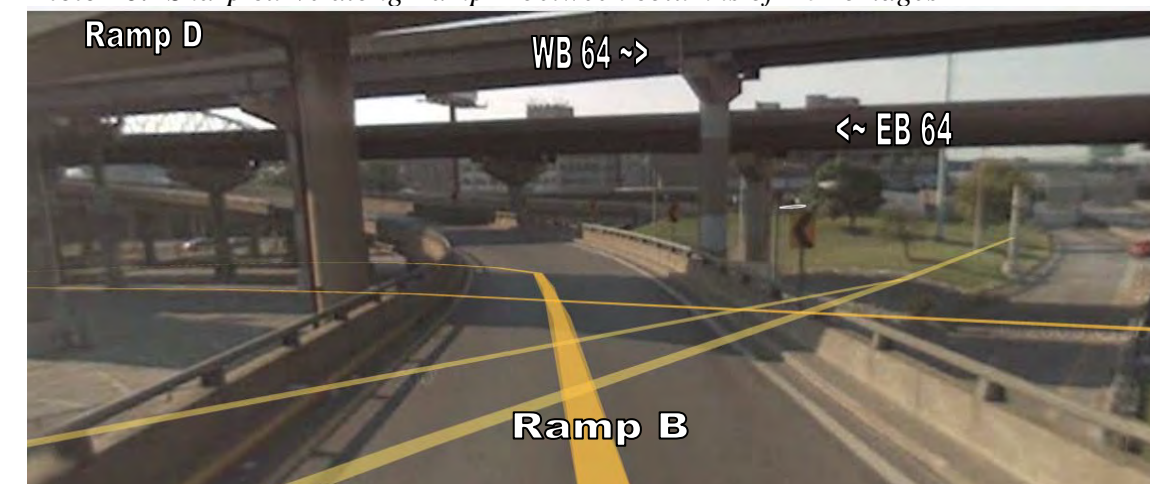
Photo 16: Sharp curve along Ramp B between columns of I-64 bridges
