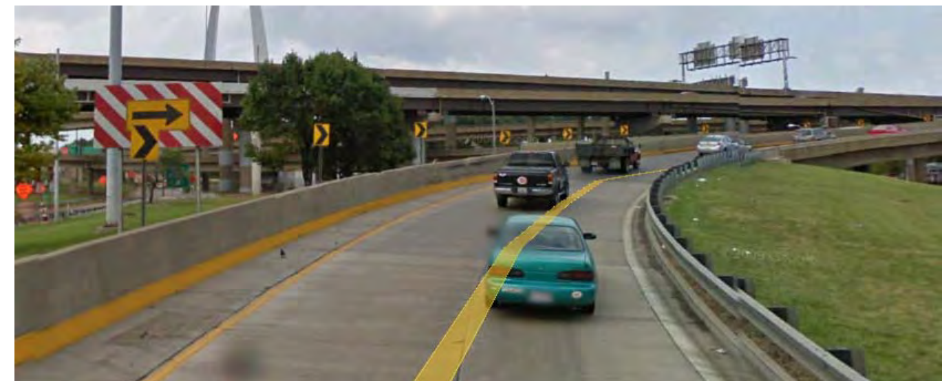
Photo 2.2: Sharp Horizontal Curve on Ramp A
