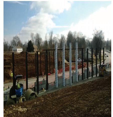
Bridge walls going up at Motherhead Road.
