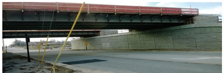
The new Hanley Road overpass.
