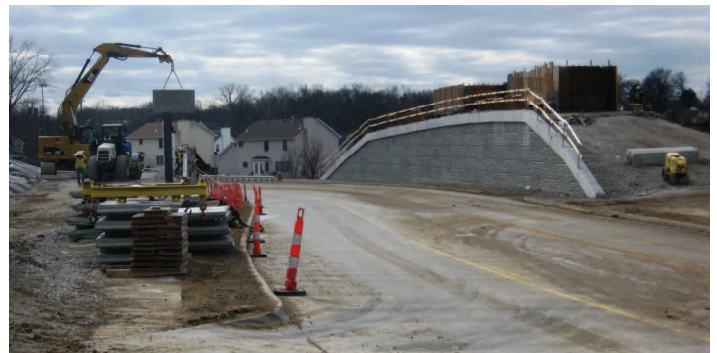
Work continues at Motherhead Road.
