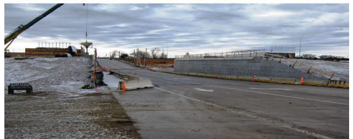
New bridge walls going up at Henke Road.
