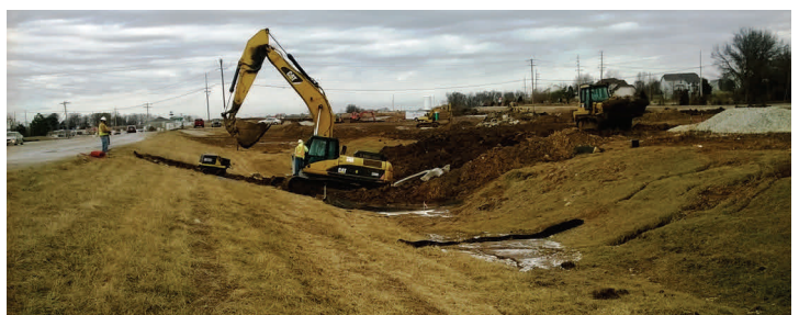
Pipe work near Bryan Road.
