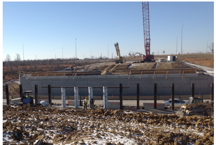
Crews are building the walls for the new bridge over Henke.
