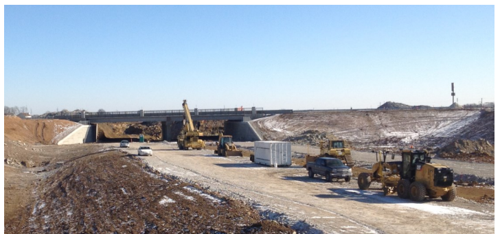
Crews are working on base rock for 364 under Bryan Road.
