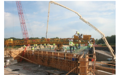
Crews poured the concrete bridge deck at Gutermuth Road on August 15.
