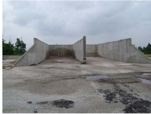
Concrete Salt Bay
