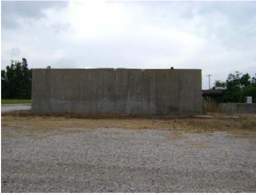
Concrete Salt Bay
