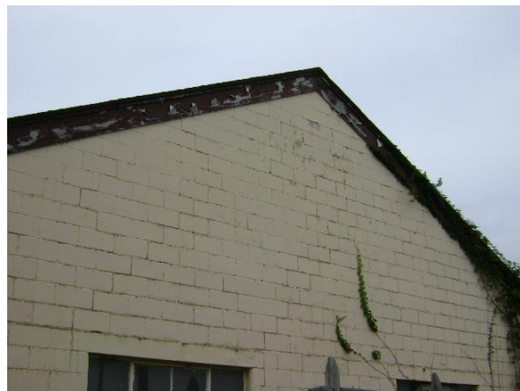
Maintenance Building/East Side
