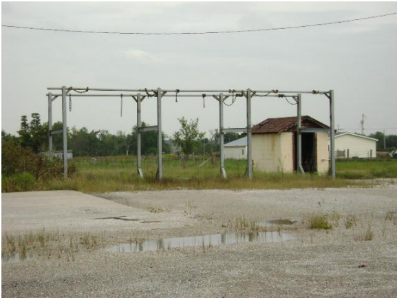
Salt Spreader Storage Rack
