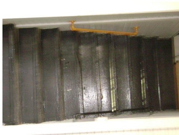
Stairs to Loft/Mezzanine
