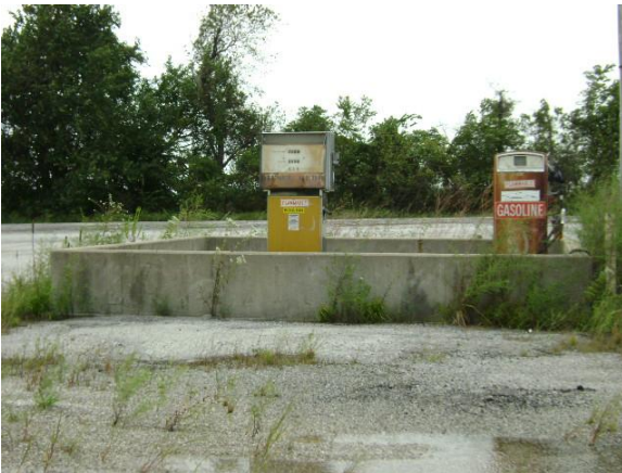
Gas Pumps/Fuel Containment Area
