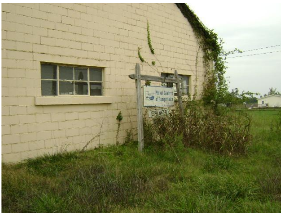
Maintenance Building/East Side
