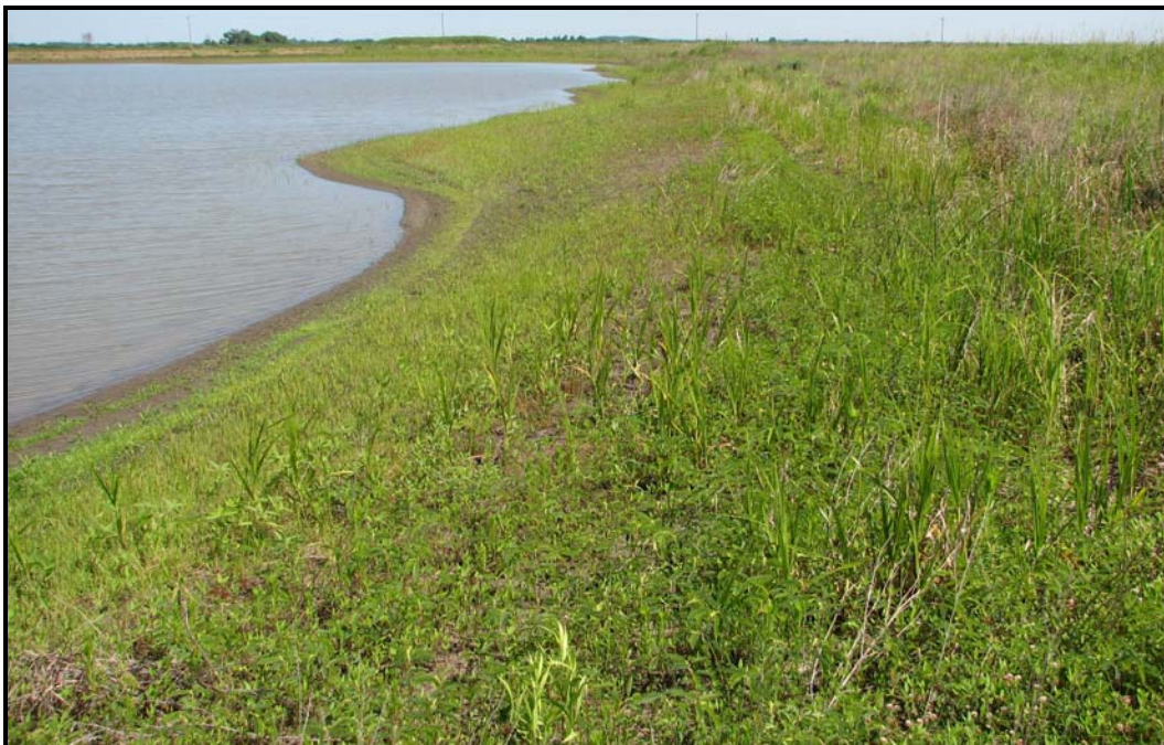
Photo 20. Eastern leg of site, facing north. (June 13, 2006)
