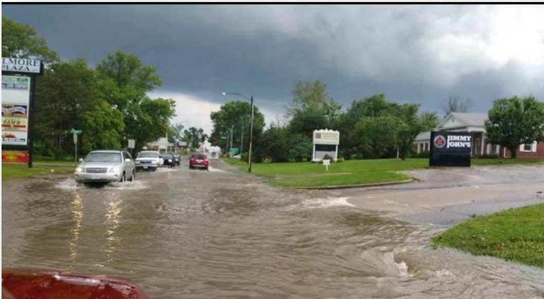
Figure 5: Flooding on U.S. Business 63/Baltimore Street after a typical rain in Kirksville, Missouri, 2015
