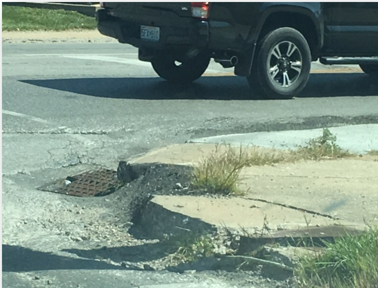
Figure 8: Existing sidewalks and curbs present hazardous conditions for both pedestrians and wheelchair users between LaHarpe and Illinois Streets
