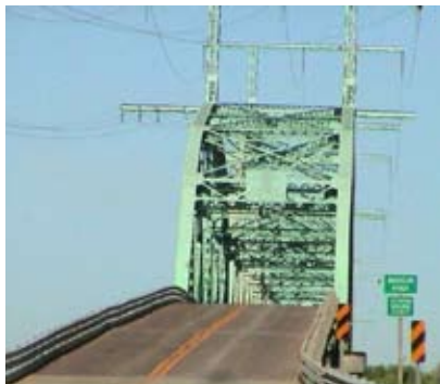
Glasgow Bridge over the Missouri River.
