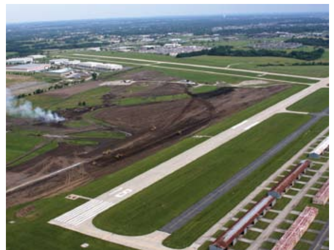
Lee's Summit Municipal Airport - East apron construction
