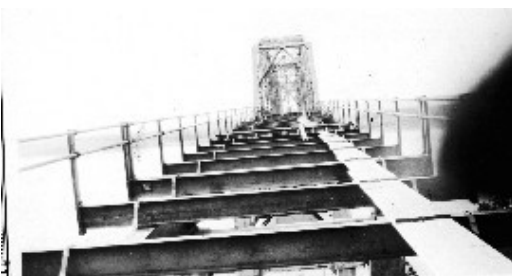
The Hermann Bridge Under Construction
