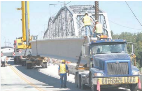
(Upper left and right) MoDOT designers check out construction on the bridge in 2006. (Bottom left) Randy Aulbur and Bob Davidson, construction inspectors for MoDOT, discuss the project. (Bottom right) The last 50-ton girder arrives in September 2007.
