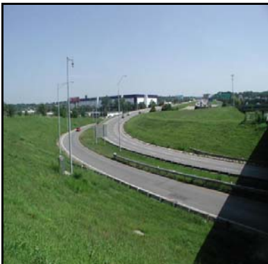
Westbound I-70 at the Benton Curve
