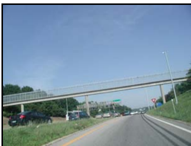
Pedestrian bridge east of Van Brunt Boulevard
