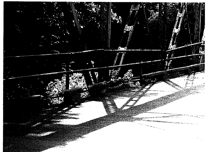
West Side Edge Barrier
