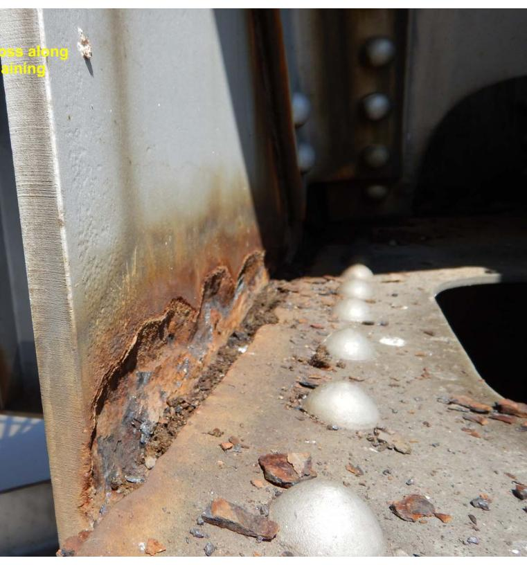
L0962 Cooper 70 9/10/15 Span 14 L16' floorbeam stringer 9 cantilever bearing with hvy pack rust
